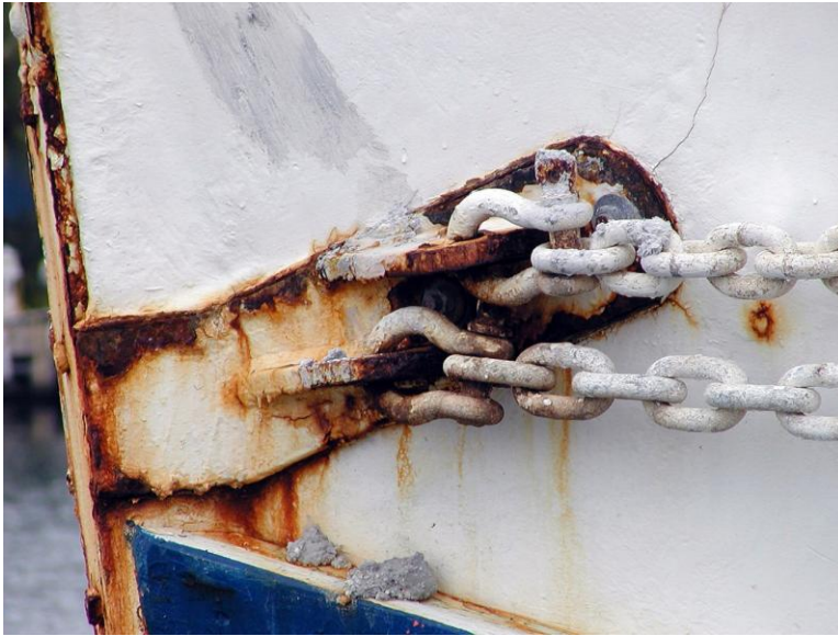
Hand-cut and -welded chain plates are rusted past worry about failure.
